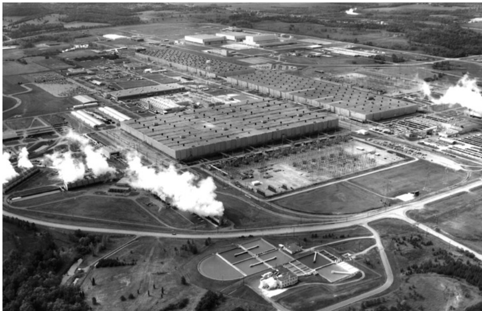
Figure 2.2. The U.S. Portsmouth Gaseous Diffusion Plant when it was operating. The three large buildings contained 1812 enrichment stages and cover an area of 0.36 square kilometers. When operating at its design capacity of 8.3 million
