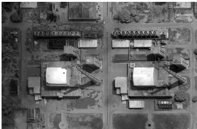
Figure 10.3. Khushab-II reactor (right) and Khushab-III reactor (left), as of September 2010.
