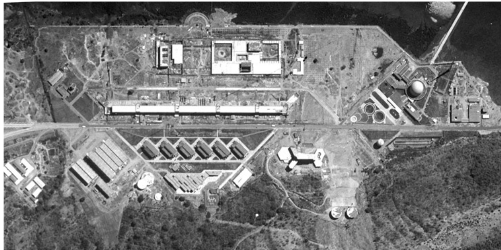
Figure 9.1. Image of the CIRUS reactor by the KH-7 reconnaissance satellite on 19 February 1966. The acronym “CIR” stands for Canada India Reactor and the “US” was added after the United States supplied heavy water for the reactor. It became critical in 1960 and its spent fuel was reprocessed at the
