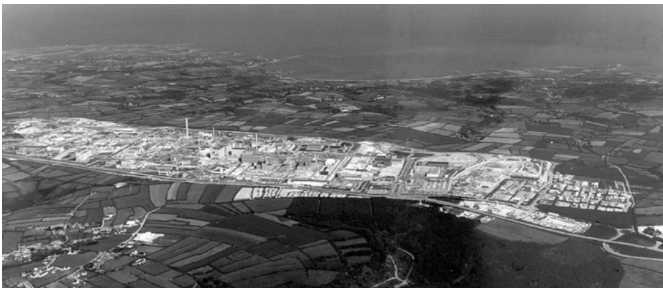
Figure 6.6. The La Hague reprocessing site. The 700-acre site includes the two reprocessing plants UP2-800 and UP3, a plutonium store, four large
