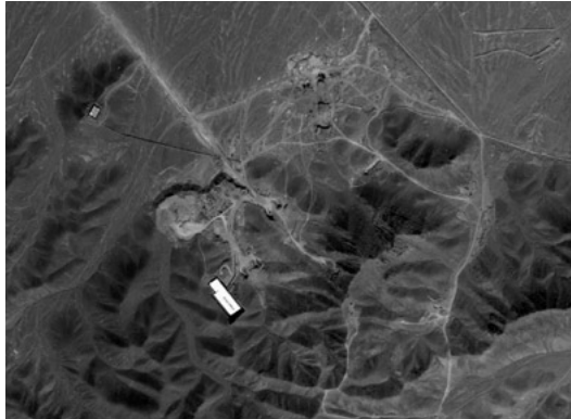
Figure 1.5. Iran's second enrichment plant (34.885 N, 50.996 E), near the city of Qom.
