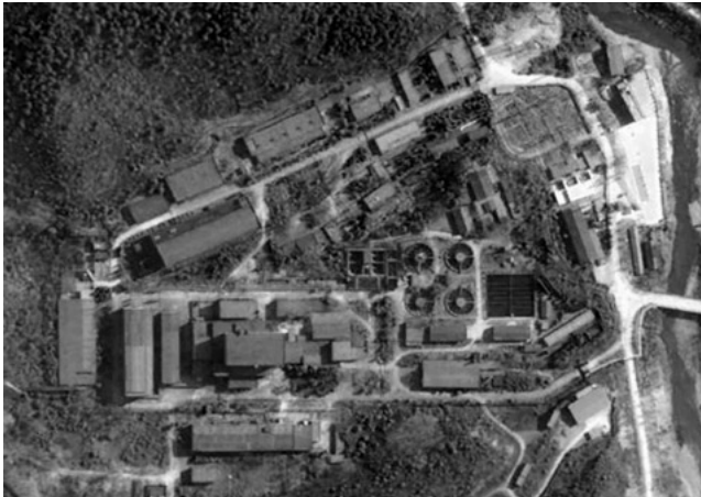
Figure 7.5. The Guangyuan reactor site, 13 February 2006 (Coordinates: 32.4956 N, 105.5901 E). Source: Google Earth.
