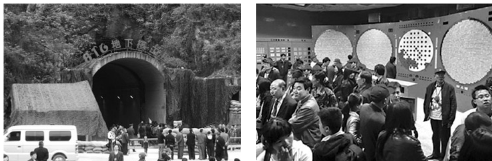
Figure 7.4. Left: Entrance to the Fuling nuclear complex. The sign in Chinese above the tunnel reads "816 Underground Nuclear Project." Right: Project 816 reactor control room. This image shows
