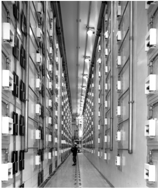
Figure 5.5. Plutonium store at Sellafield, UK. Sellafield in West Cumbria is the UK's center for reprocessing spent nuclear fuel from Britain's nuclear power stations and overseas customers. More than 100 tons of plutonium are stored at this site. Credits: British Nuclear Fuels and IAEA ImageBank.
